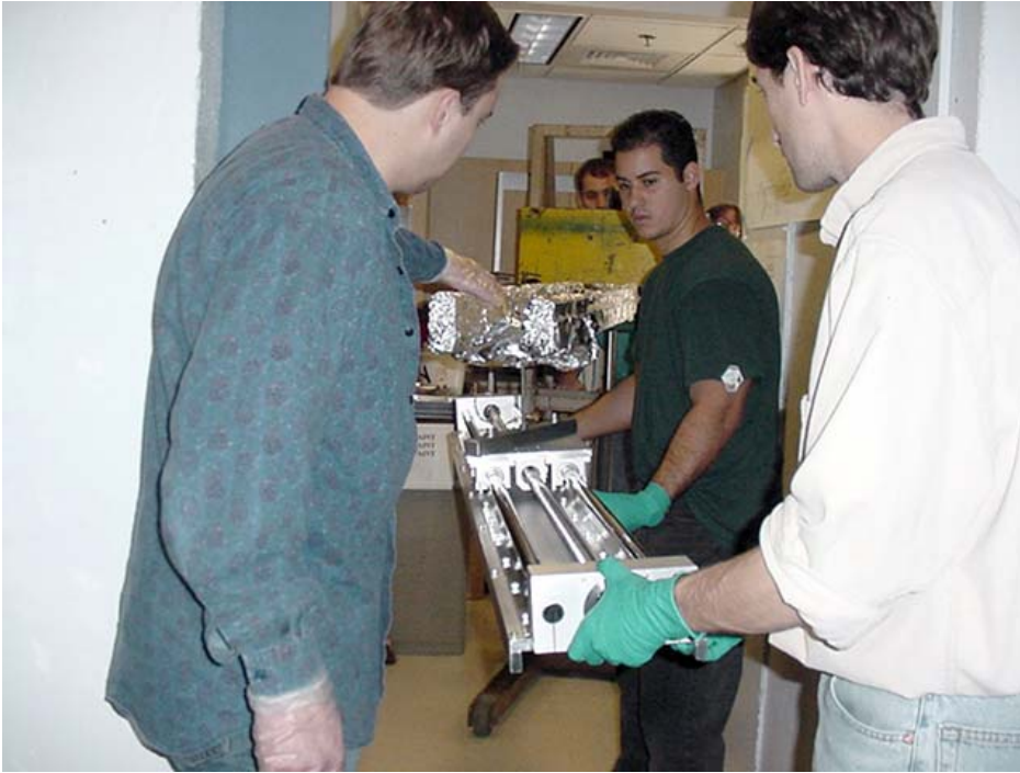
Blasini (center) helps the CHES technical crew install a 2-meter long in-vacuum optics translation stage. Tom Krawczyk is left, Chris Conolly right, and Dana Richter controlling the hand lift in rear.
